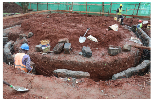
Ongoing construction at the NWST Karen Campus, Nandi Road
